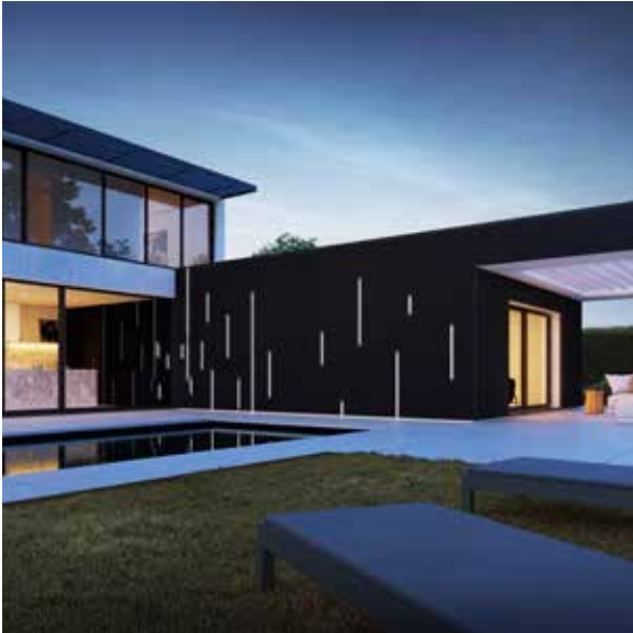
Filled with LED modules
